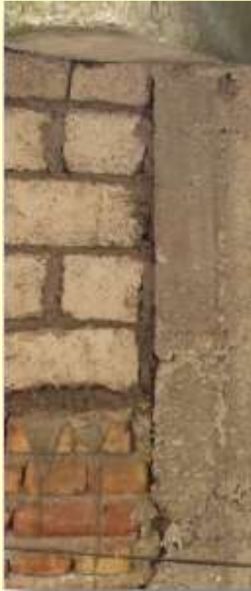
RC - Columns first, walls later
