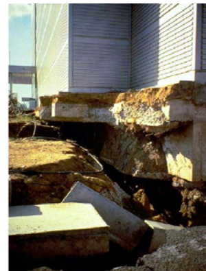
Settlements and tilting of the buildings
