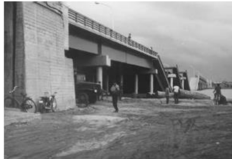
Fig. 24.64 Fallen Showa Bridge crossing Shinano River (Department of Civil Engineering, University of Tokyo)
