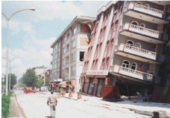
Bearing capacity failure of a building after Izmit EQ, 1999
