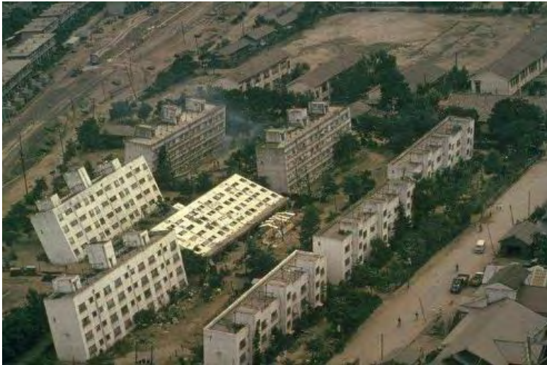
Loss of Bearing Capacity, Tilting of Kavagishi-cho Apartment Buildings, 1964 Niigata
