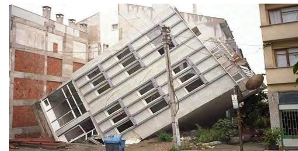
Settlements and tilting of the buildings
